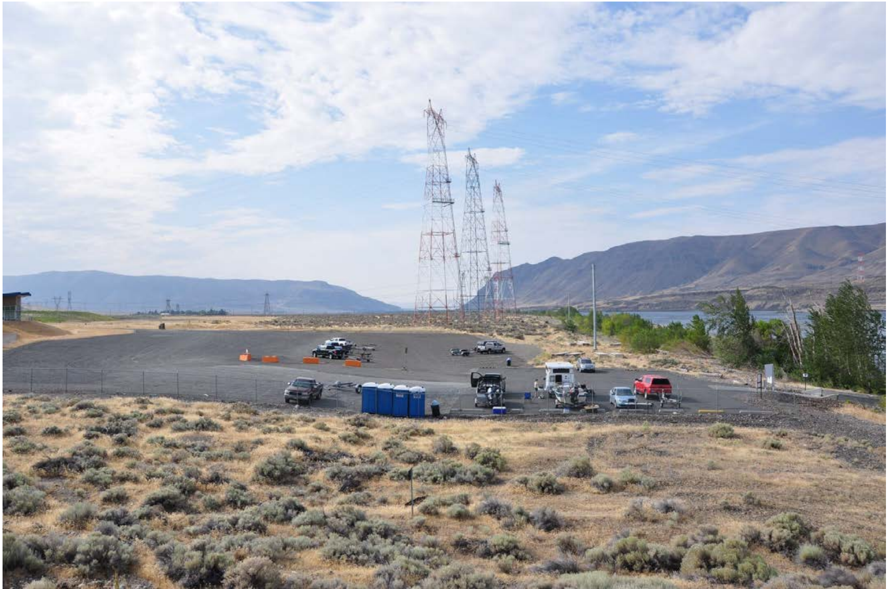
Wanapum Dam Lower Boat Launch
